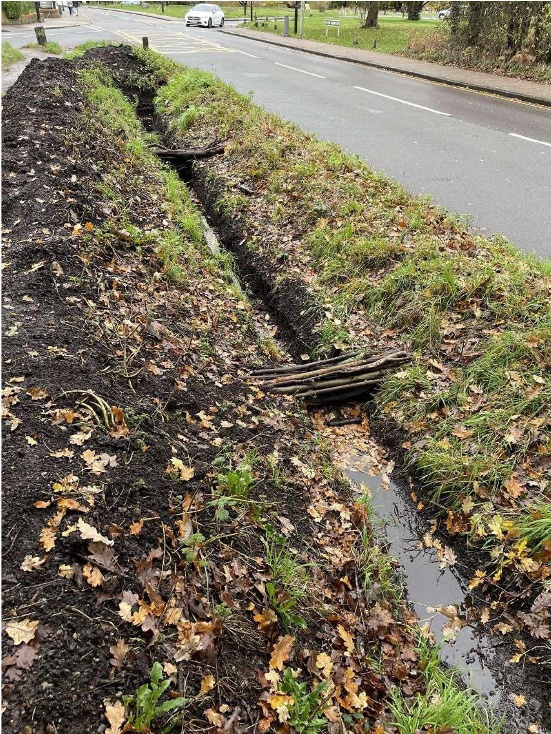
As this photo shows, the logs slow down the water, and the silt settles out before it reaches the drain.
